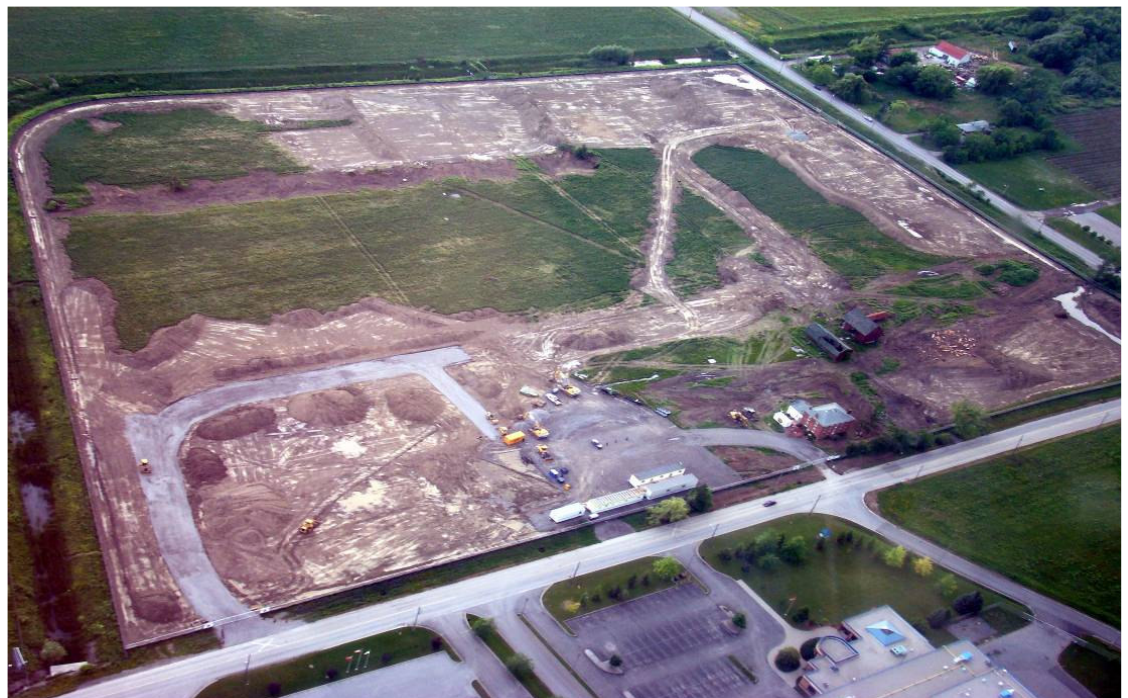
An aerial view of the site at First Street and Fourth Avenue, taken June 21, 2009
